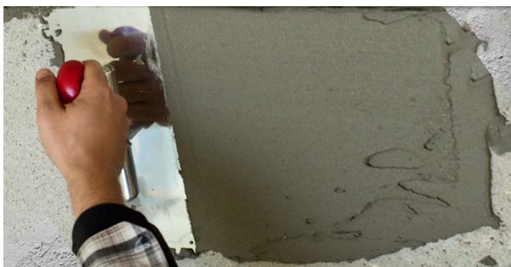
Fig. 2: Flat screed the adhesive.
