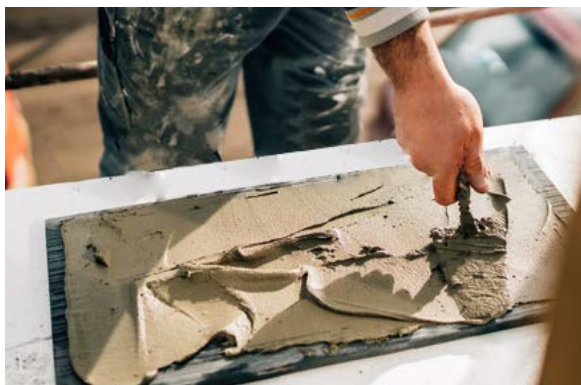
Fig. 3: generously back butter the stone.
