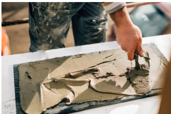
Fig. 3: generously back butter the stone.
