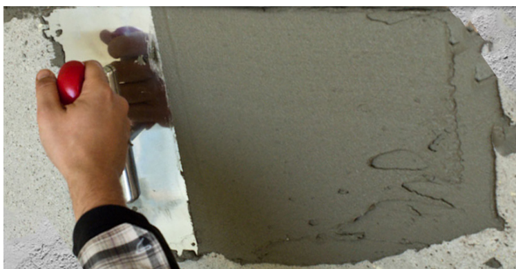
Fig. 2: Flat screed the adhesive.
