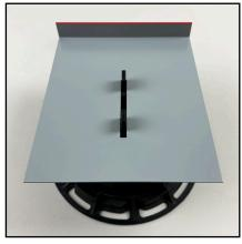
**Step 4:** On the upstand of the pedestal bracket run a bead of Ardex CA20P Adhesive Silicone for the profile edge to attach on to.
