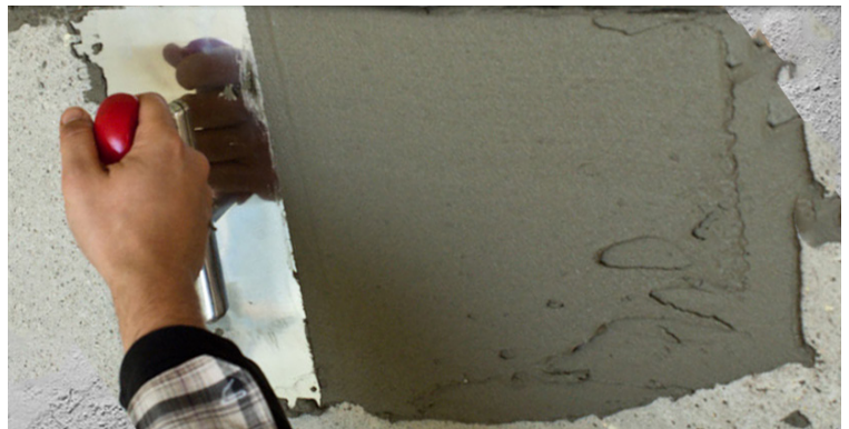
Fig. 2: Flat screed the adhesive.
