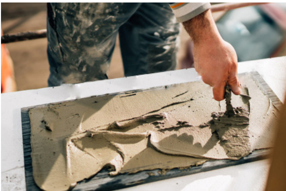
Fig. 3: generously back butter the stone.
