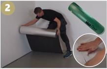
• Lay Maxplus Premium IXPE Underlay and ensure the sheets are sealed together using the self adhesive strip on the back. Tape all sheet joints with a 50mm P/E Tape Such as Davco Bond Breaker Tape.
