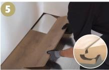
• Match the long edge first, keep an angle of 20° - 30° when inserting. Slowly slide flooring over to line up with the short edge.
