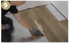
• Measure and cut next the plank to the required size and ensure the perimeter gap is maintained. Any off-cuts (min 300mm) from one end can be used to start the new run which ensures a natural random joint structure. Please also ensure on installation that each row is staggered so that no joints are closer than 300mm (we recommend a minimum of 1/3 of the full length).
