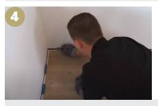
• Provide a 10mm expansion gap between the Max Floor and your walls or fixed objects. This is allowance for the minimal expansion rate which is -/+ 0.1% average. When skirting is installed, ensure there is an expansion gap beneath.
