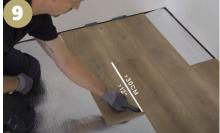
• Measure and cut next the plank to the required size and ensure the perimeter gap is maintained. Any off-cuts (min 300mm) from one end can be used to start the new run which ensures a natural random joint structure. Please also ensure on installation that each row is staggered so that no joints are closer than 300mm (we recommend a minimum of 1/3 of the full length).
