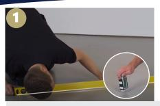
Check that the substrate is level and free from moisture to confirm suitable for installation. Consider need for moisture seal or P/E sheeting.
