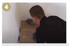
• Provide a 10mm expansion gap between the Max Floor and your walls or fixed objects. This is allowance for the minimal expansion rate which is -/+ 0.1% average.
