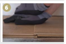
• Slowly drop the plank down and click the short edge down with your hand. Do not use a mallet or pulling iron, the flooring will easily click together.
