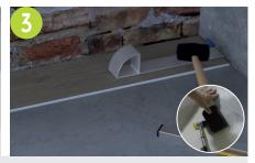
• Use a pulling iron and mallet to gently tap the short side into place, then use a tapping block to fasten the locking system on the long side.
