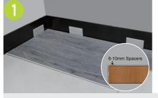
• Provide a 6mm - 10mm expansion gap between the Max Floor and your walls or fixed objects. This is allowance for the minimal expansion rate which is -/+ 0.1% average.
