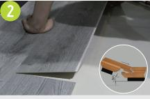
• Match the long edge first, keep an angle of -/+ 20° when inserting. Make sure the short sides are as close together as possible, e.g. 10mm or less.
