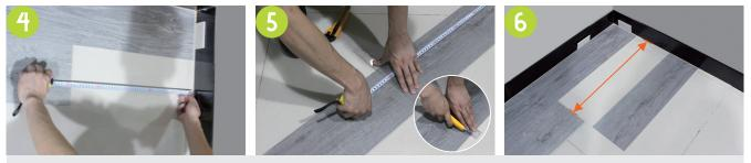
• Measure and cut the plank to the required size and ensure the perimeter gap is maintained. Any off-cuts (min 300mm) from one end can be used to start the new run which ensures a natural random joint structure. Please also ensure on installation that each row is staggered so that no joints are closer than 300mm.
