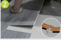
• Match the long edge first, keep an angle of -/+ 20° when inserting.
