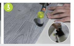
• Use a rubber mallet to gently lock the short side, then use a tapping block to fasten the locking system.
