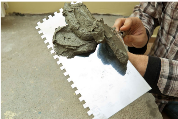
Fig. 1: Adhesive on trowel to be burnt into the substrate.
