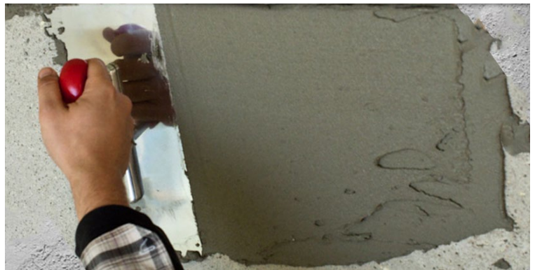
Fig. 2: Flat screed the adhesive.
