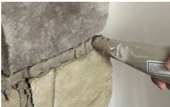
Fig. 4: Ensure all joints are evenly filled with adhesive - no gaps.
