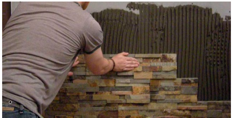
Fig. 4: Bed each piece of stone, letting adhesive come through.
