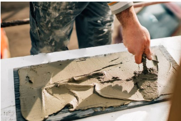
Fig. 3: generously back butter the stone.
